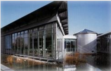
Zuken GmbH European Headquarters Munich, Germany
